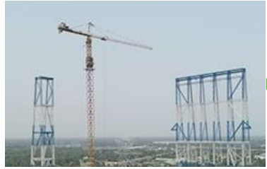
Test Station and R&D Center
