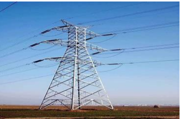
Power Transmission Tower
