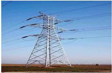
Power Transmission Tower
