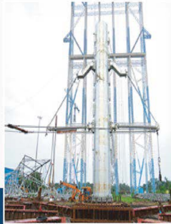
400kV Composite Insulated X-Arm India (CICA)
