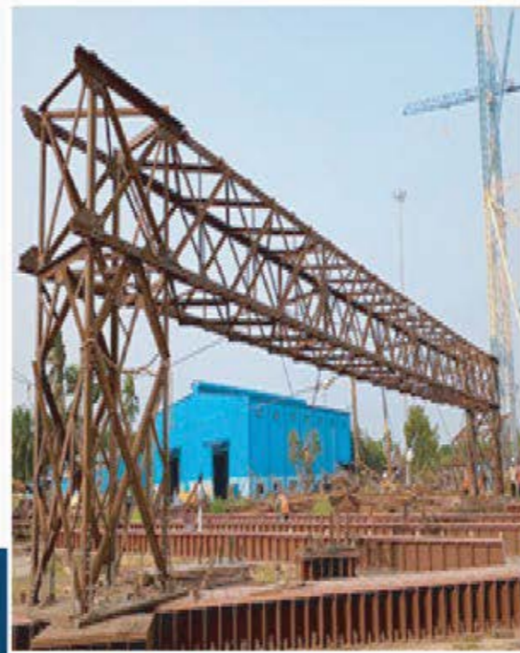
220kV Substation Beam India
